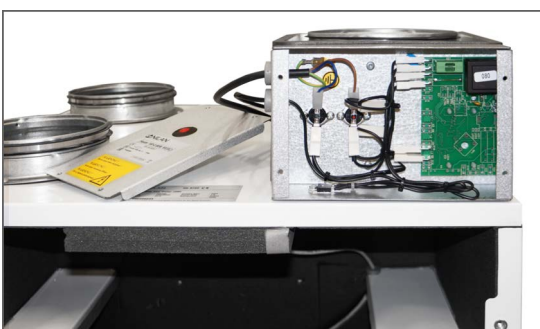
7. The power supply cable is pre-mounted in the unit and the preheating surface connected with Phase (F), Zero (N) and Ground (J).
