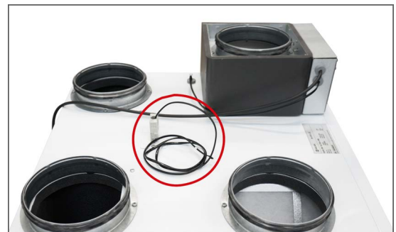
6. The T1 sensor is pulled from the 8-pole outlet into the outdoor air duct (30 cm before the preheating surface).
